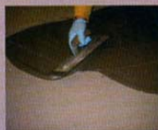
Sika® Primer MB is a roller applied damp-proof membrane
